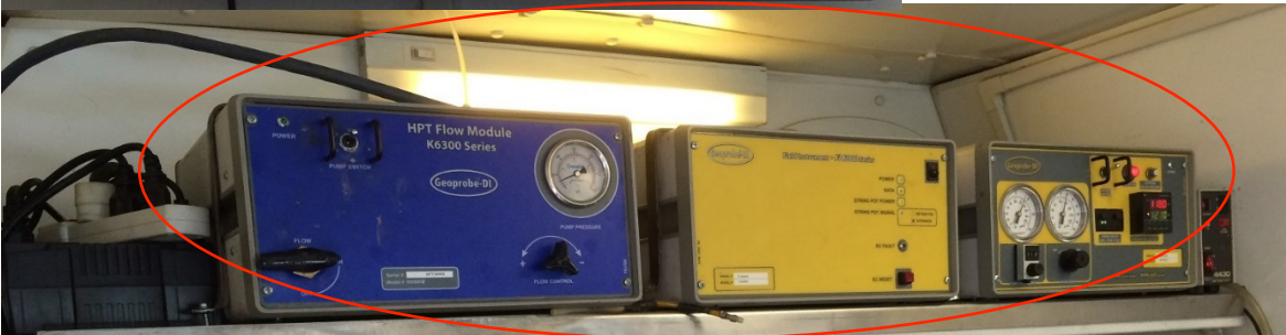
Trunk line controls
